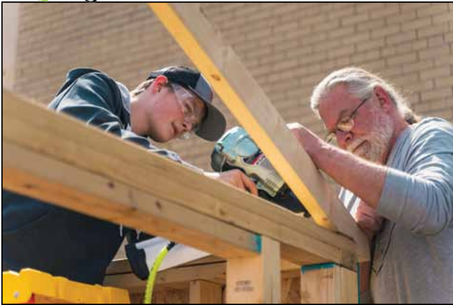
Dahl and Miles Hooper work on the shed.
